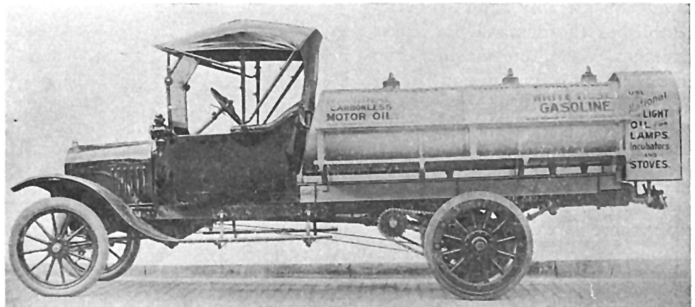
Converted chassis equipped with a tank body for distributing oil. This is a very practical and economical equipment.
